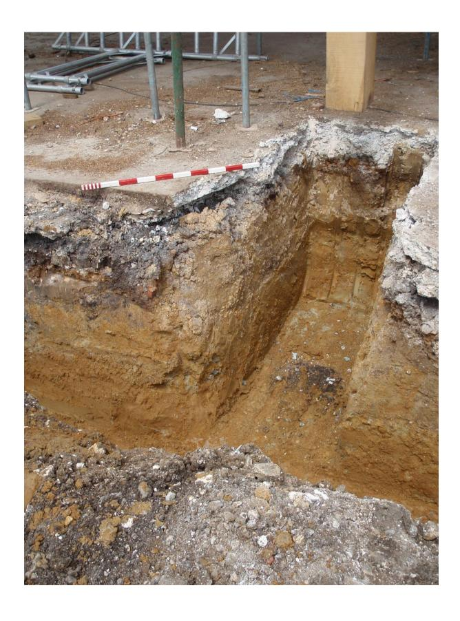
Plate 5. Mid 19<sup>th</sup> century brick foundations on the south-east side of the barn
